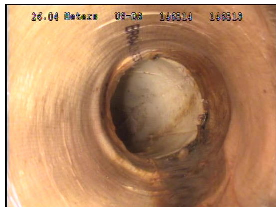
Figure 12: View inside the lateral connection
