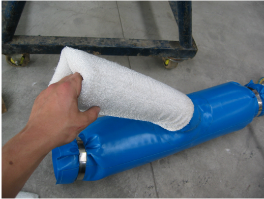
Figure 6: Inverted liner inside the lateral
