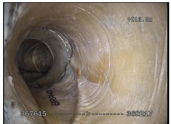
Figure 9: LJR with a small wrinkle caused due to RI
