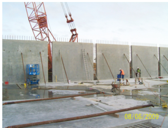
Figure 2: Precast Panel Installation
