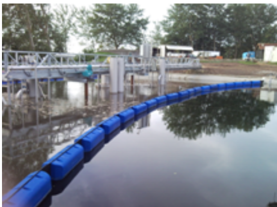
Figure 5 : CWSBR® Control Bridge and Hydrosail separating activated sludge zone from clear water zone
