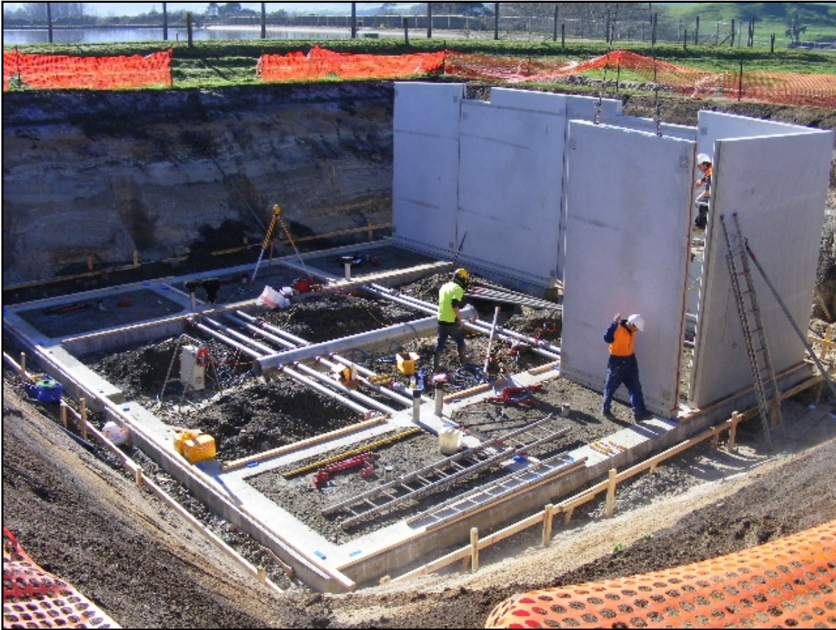
Figure 12- Membrane Filtration Plant During Construction
