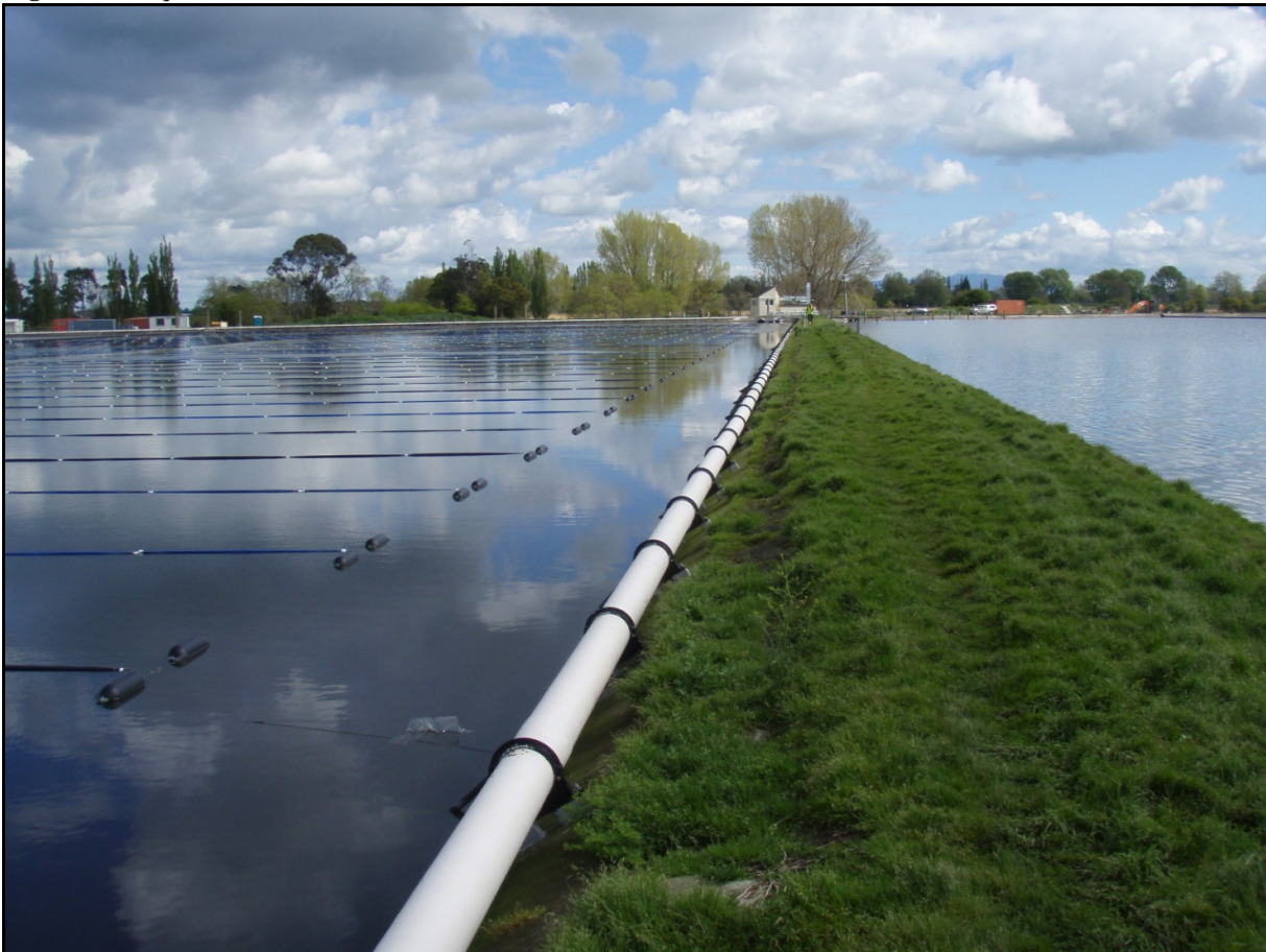
Figure 6 – Aquamat Installation at Matamata WwTP
