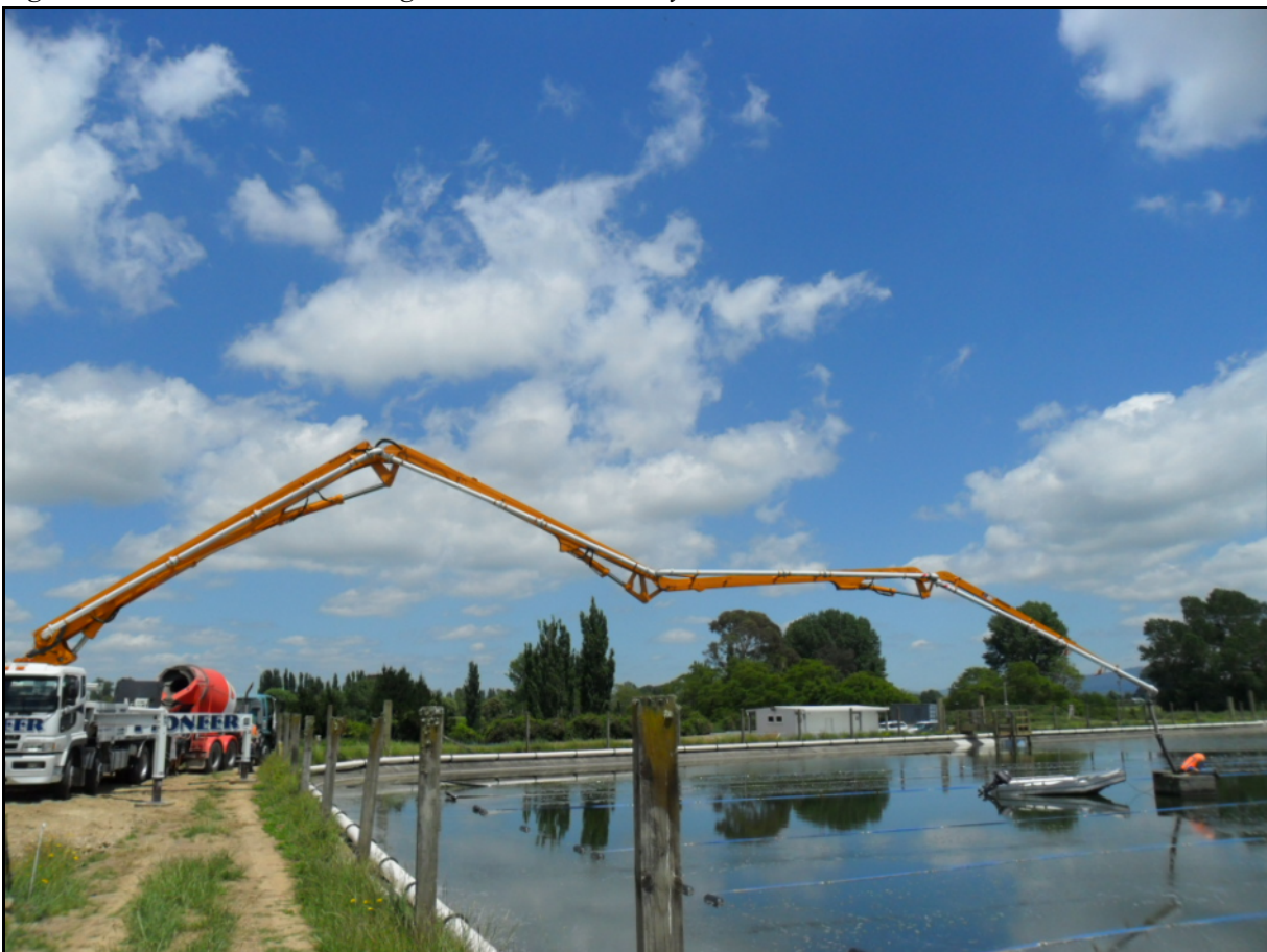
Figure 11 – Construction in Progress within Secondary Pond
