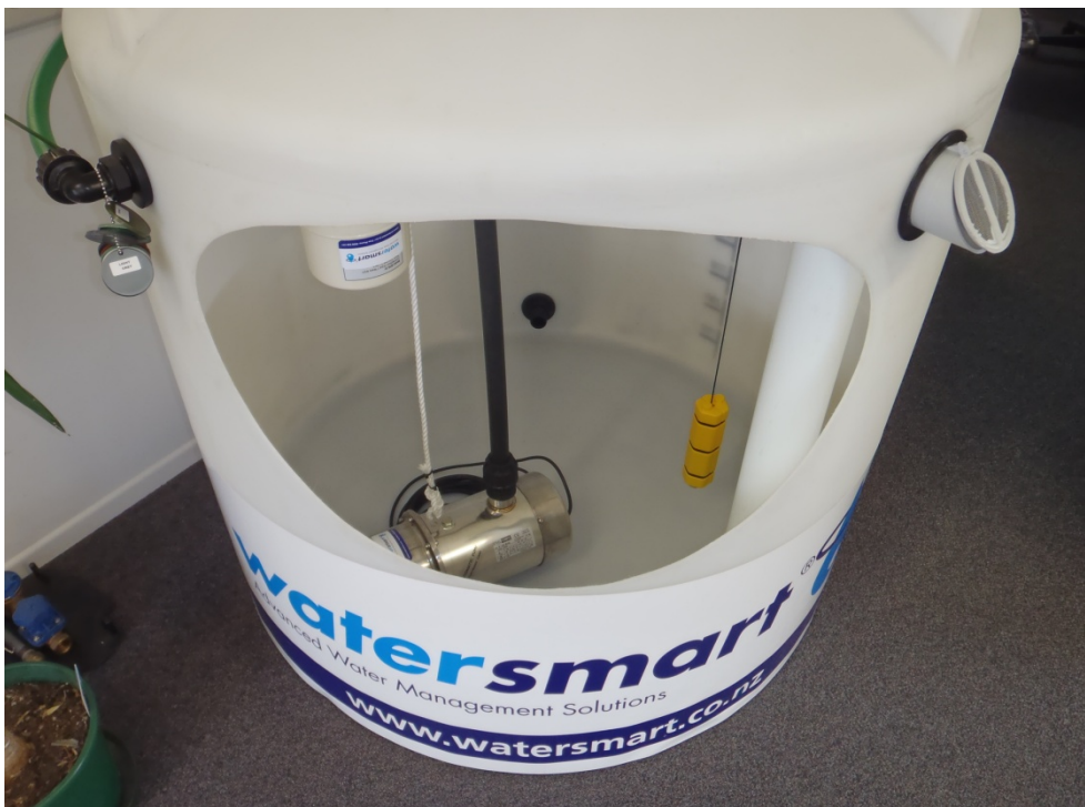
Photograph 3: Hush pump example showing pump in tank
