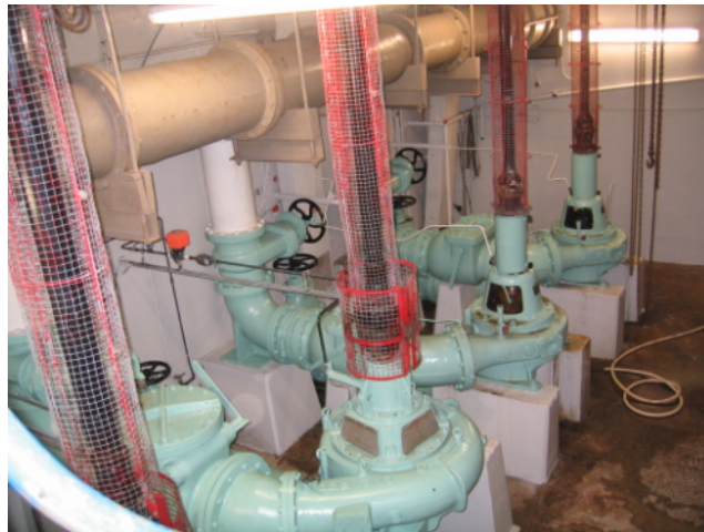
Photograph 2: Original pump station dry well
