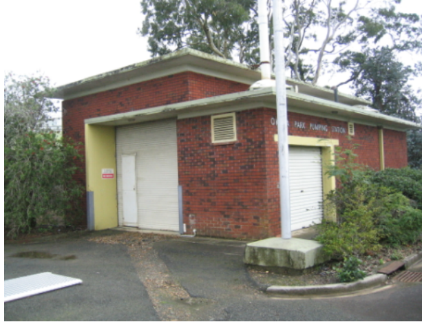
Photograph 1: Original pump station building
