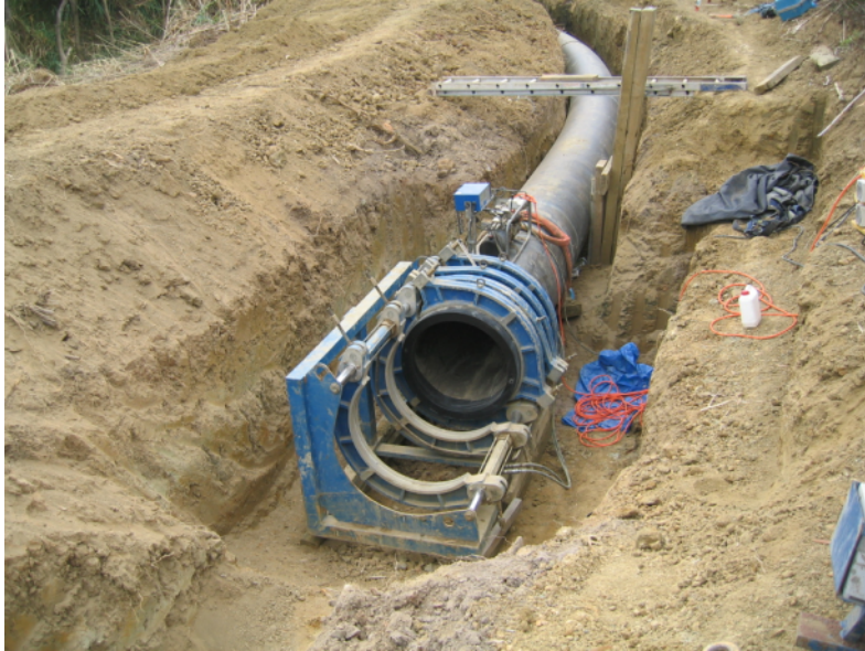
Photograph 6: Rising main under construction
