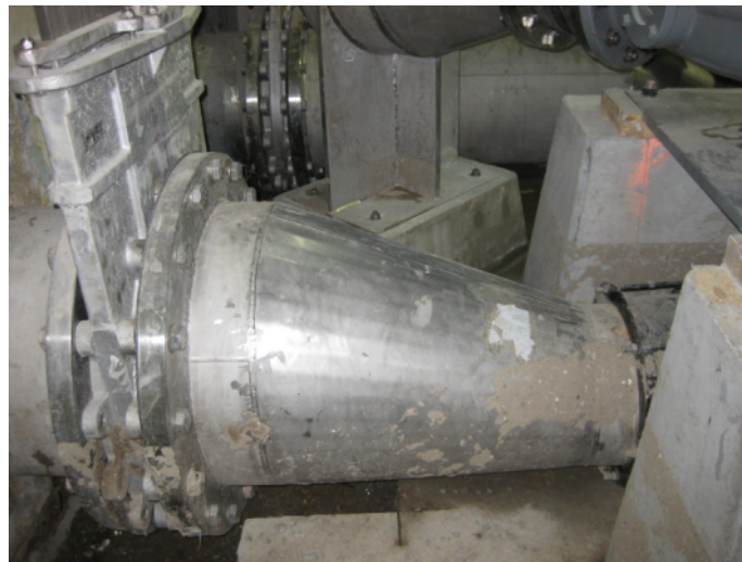
Photograph 3: Eccentric taper and flanges cut into floor
