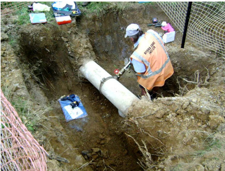
Figure 3-2 Recovery of an AC Core Sample
