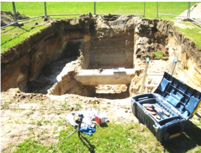
Figure 3-1 Shows a Well-Planned Excavation
