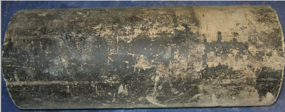
B1-1: Typical external view of an Everite pipe. Approx 50% of the bitumen coating is remaining, however, the CT scan confirmed that it was providing little to no protection against deterioration.
